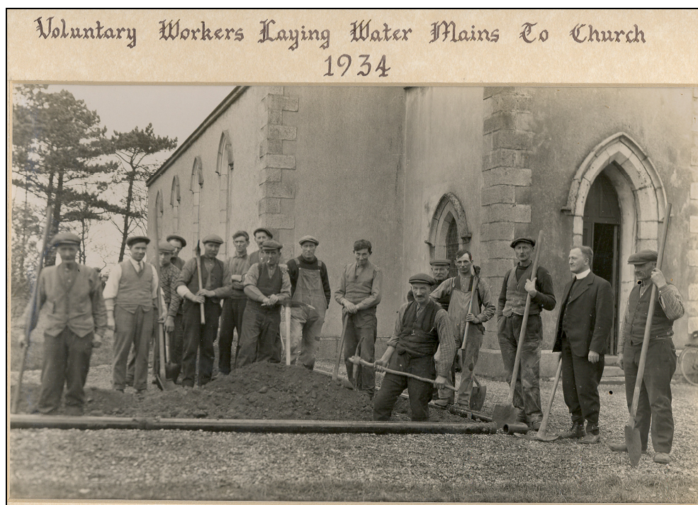
Plate Two: Photograph in possession of Kilhorne Church showing excavation of trench to accommodate water pipe (1932). The photograph depicts (from left to right) John Moore, John Cowden, Jim Arnett, William Wiggins, Frank Moore, Thos Mayhew, James White, Jack Gibson, Robert Little, Cecil Gordon, Jimmy Young, Wm. McConnell, Johnny McKibben, Wm. McMath, Rev. T.B. Lyons and Tom Cooper. The 1934 date on the photograph is difficult to reconcile with the pre-March 1932 date recorded in the contemporary published accounts of the excavation of the trench for the water pipe and the concomitant discovery of burials (i.e. Berry and Nolan 1932). It is reasonable to assume that the caption was added later and is incorrect. Photograph kindly supplied by the Reverend William Press.
