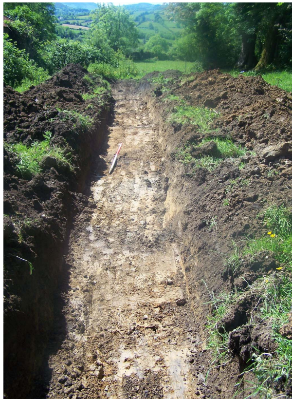
Plate Four: Trench One, looking south
