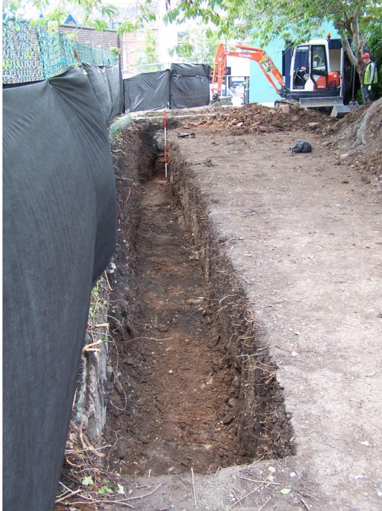
Plate 11. The cable trench during excavated in 2011. Shot taken from north.
