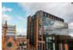
2 The Main Site Tower
